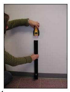
**1-** Using a stud finder attach bottom section of True Plumb to a stud. If base molding is over 1/4" thick the bottom part of the True Plumb must be mounted above base molding. Note: When mounting to a concrete wall use a 1/4" masonry bit and expanders provided.
