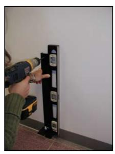
**2-** Use a level and mount the bottom section with two screws provided.
